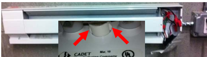
Figure 6. Adjusting a tamper-resistant thermostat. Once the faceplate is open, the plastic cover may be removed by pinching the plastic tabs (see red arrows in inset photo).
